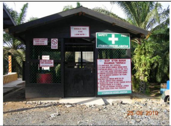
Storage areas for the chemicals at the Tangkulap estate
